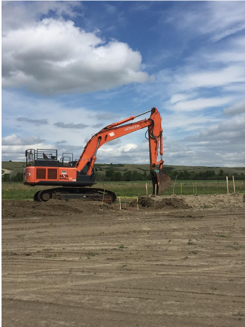
Excavator removing roach from ROW, preparing to dig for pressure tests.
