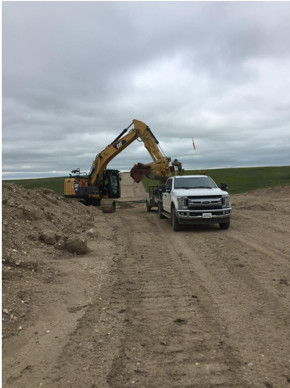
EXCAVATOR LOADING SNOW FENCE, POSTS AND T-BAR.
