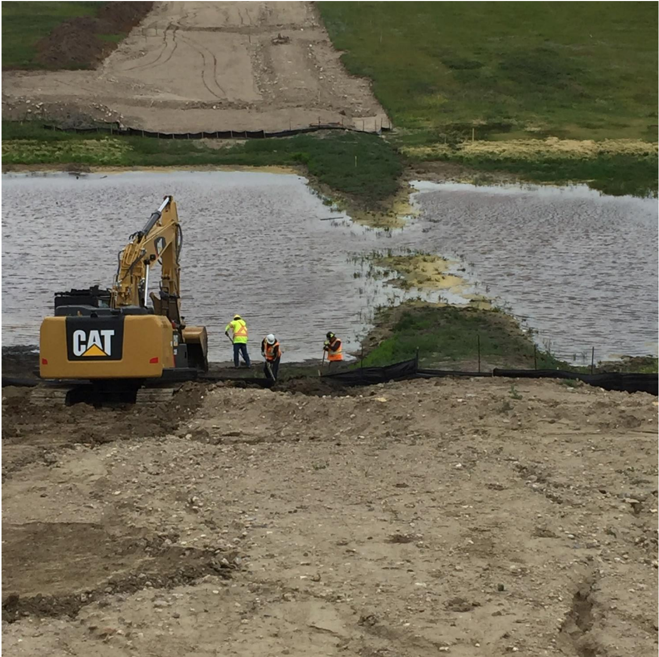
Deficiency crew working down at watercourse cleaning sediment.
